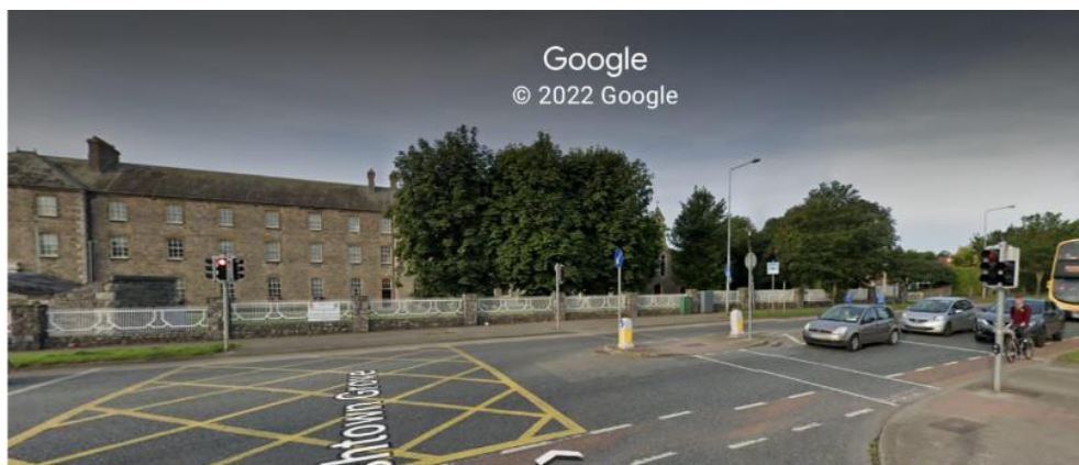
Pedestrian island at junction of Navan Road and Ashtown Grove - Surface Photo (Google Maps)
